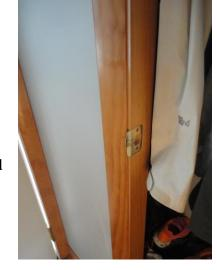
19. The original wood cabinets were modified to create room for the dishwasher. The appliance insulation is visible from the cabinet interior. The side of the cabinet should be closed off to prevent stored items from falling under the dishwasher, to keep the insulation intact, and keep pests out of the cabinet.
