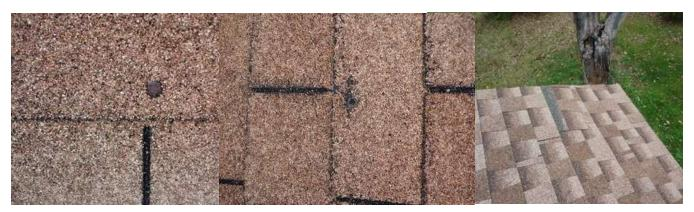
28. There is moss on the front porch roof, and on the North slope of the garage roof. A solution of bleach and water will kill the moss and it will sweep of easily when it's dry.
