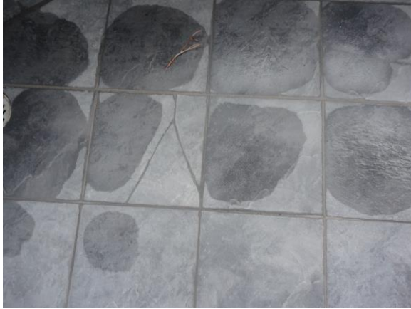
Broken tile on left, loose one on right. Near drain at the round section.
